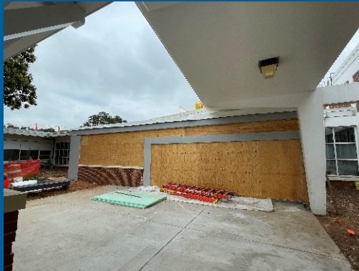
Air Barrier applied on exterior of security vestibule
