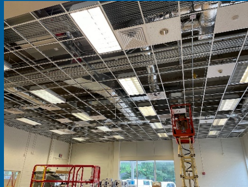
Ceiling Grid and Tile install in Cafeteria Area
