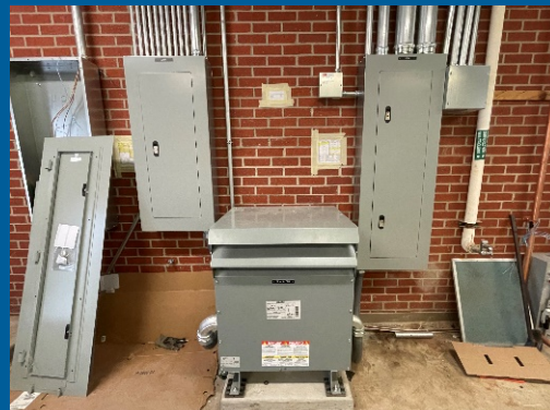
New transformer and switchboards installed
